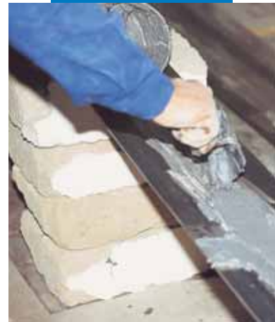
Application of Adesilex PG1 on metal sheet
