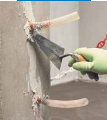
Fixing injection tubes and sealing cracks for structural consolidation
