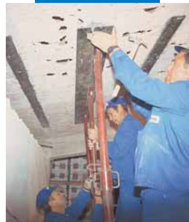
Placing metal sheet for structural reinforcement
