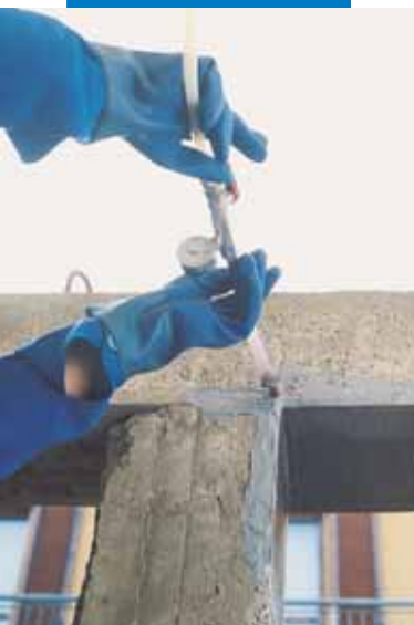
Column clad with Adesilex PG1
