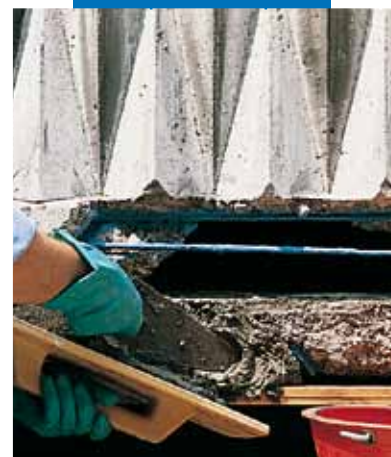
Repairing a balcony with Mapegrout T40
