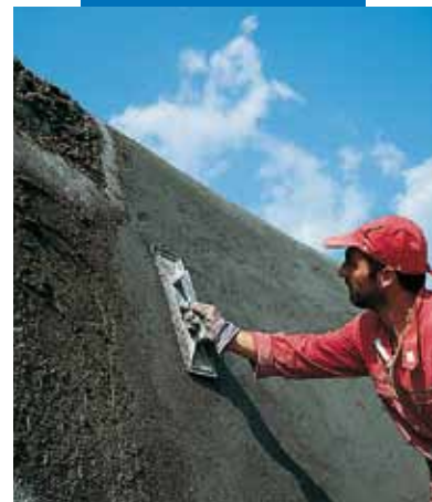
Finishing of Mapegrout T40
